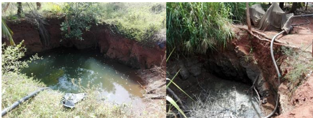
Fig. 5.6: Unprotected wells which are used for agro based activities, Thanthirimale Source: Field survey (2016)
