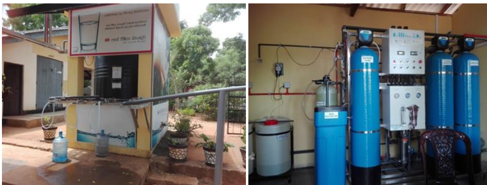
Fig. 5.10: Water purification station and the equipment kept inside the station Source: Field survey (2016)
