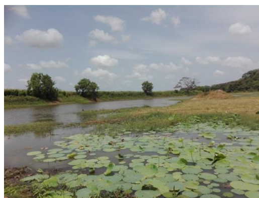
Fig. 5.9: Reservoirs in Thanthirimale (Kuda Malmaduwa Tank) Source: Field survey (2016)
