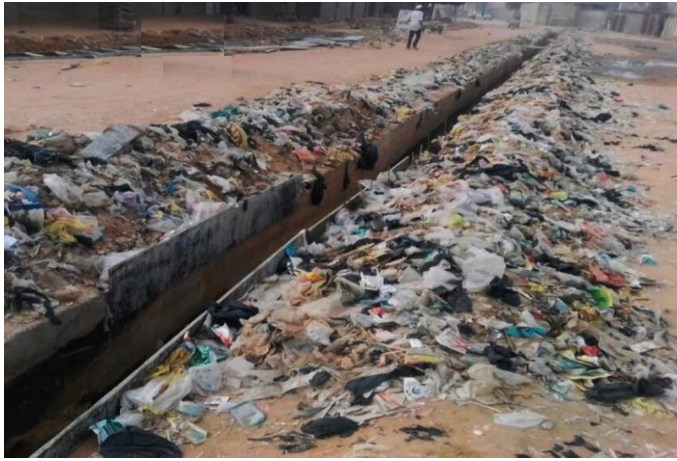
Fig. 5: Open Drainage Refuse Dump in Hotoro
