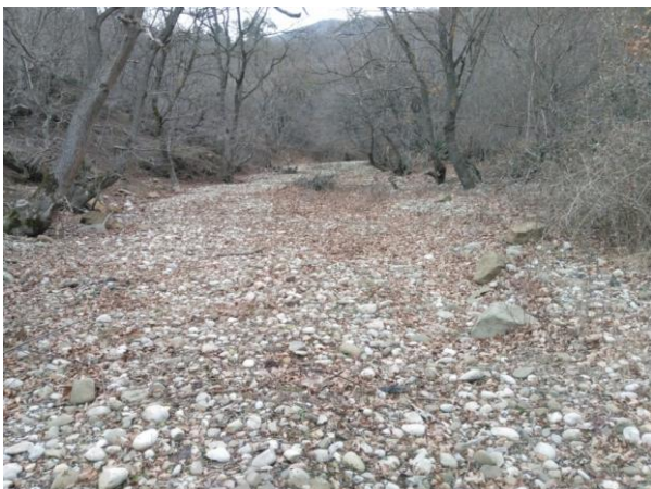
Photo 2: The sediment debris flow material in the bed of Jokhtaniskhevi
