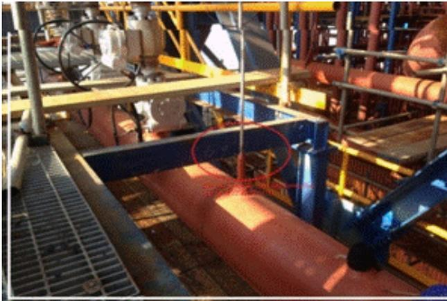
**Fig. 1:** Welding dust shields of the boiler roof section between 304L austenitic stainless steel and carbon steel
