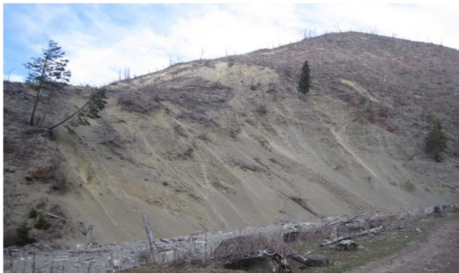
Photo 2. Active erosion processes.
