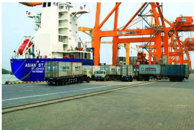
Fig. 3: Crane system of Hai Phong port
