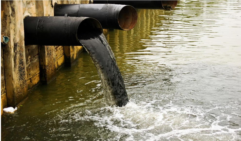
Fig. 2: Oil pollution from waste water
