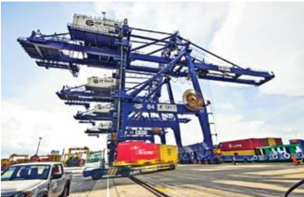
Fig.3: Crane system of Hiep Phuoc port
